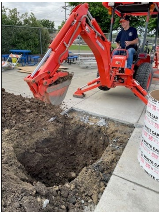
May Nissen Shade Structure
