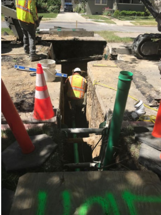
Trevarno Road Sewer Construction
