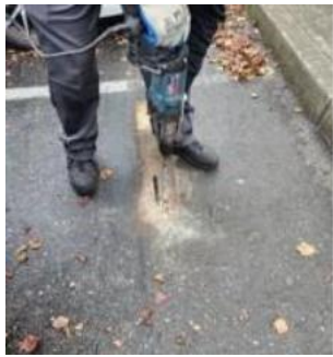
Parking lot bump repair at ESS parking lot
