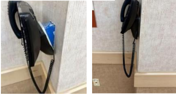
RLCC Phone Wall Repair
