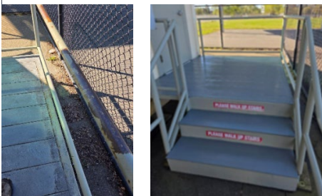
Repaint handrails at Smith ESS
