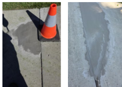
RLCC pathway tripping hazard repair
