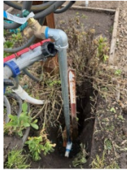
CG irrigation replacement
