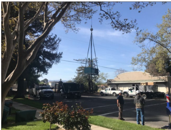
Trevarno HVAC Installation
