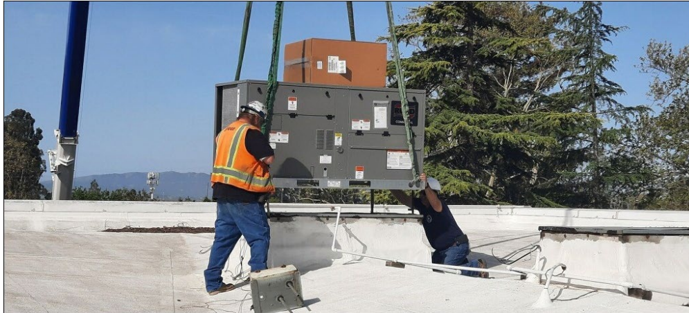
Trevarno HVAC Installation
