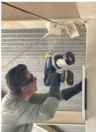
Rodeo Stadium Improvements
